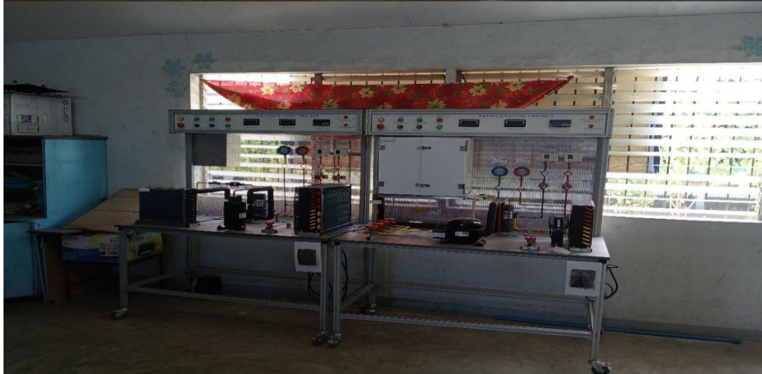
(f) Steam Boiler, Steam Turbine, Refrigeration
